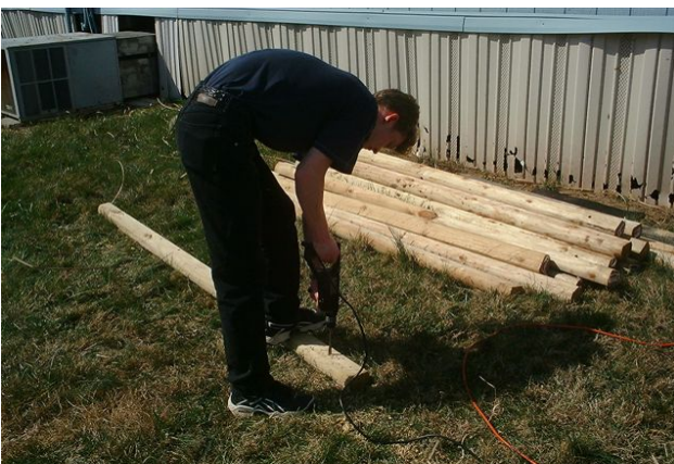
Drilling holes...allot of holes.....
