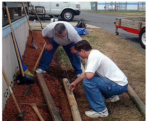
Seniors laying new timbers.....
